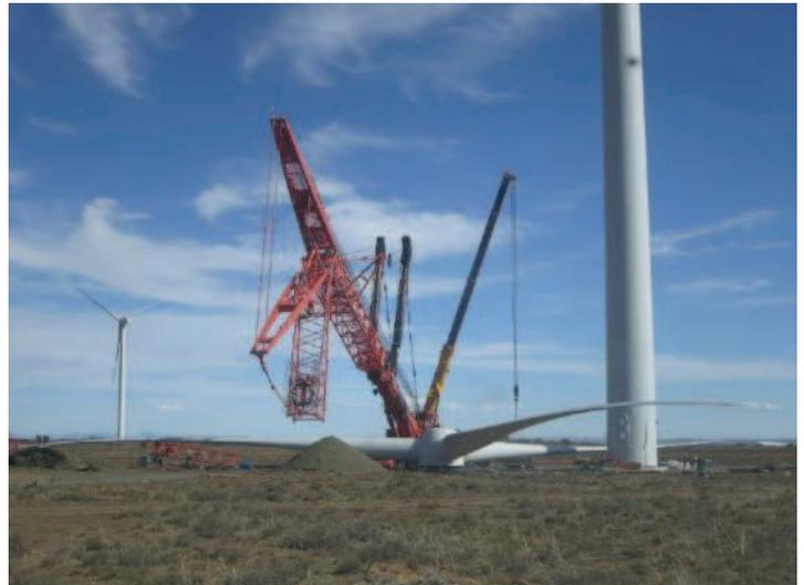
Placing a tower in position prior to lifting the hub with the fan blades already in place. A special crane is used to take the hub to the top of the tower, where it will be lined up and fitted under the guidance of a perched engineer, wearing a hard hat and a parachute, we hope.
